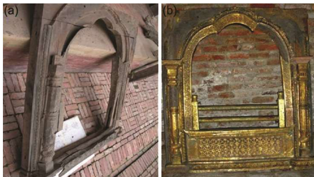
Fig. 2 — Photos of 17 th century gilded window from Royal Palace Patan, Nepal (a) before and (b) after conservation.
