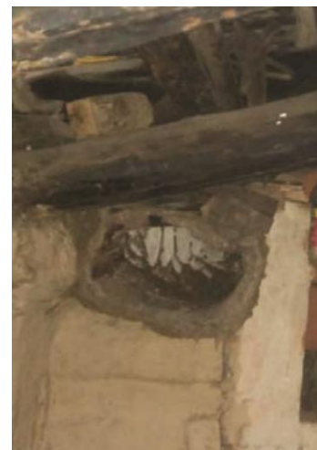
Fig. 1 — Outer view of wall hive
